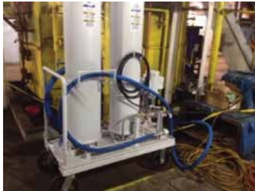
(HILCO ® model 36118-53040100 installed on a customer's 2,800 GAL EHC Reservoir)
